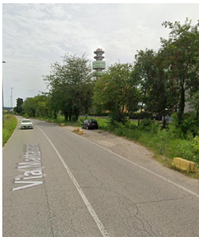
La zona Telecom in Via Mattarana
